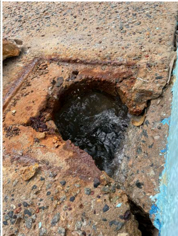
Cracks in inspection pits behind pool end wall
