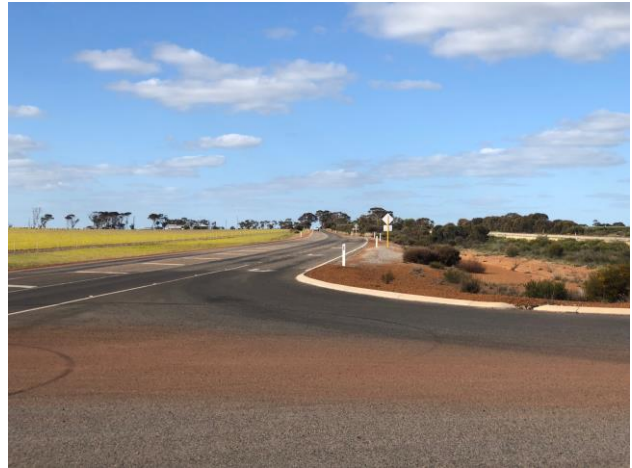
Sight distance available Goomalling Wyalkatchem Rd (looking east)
