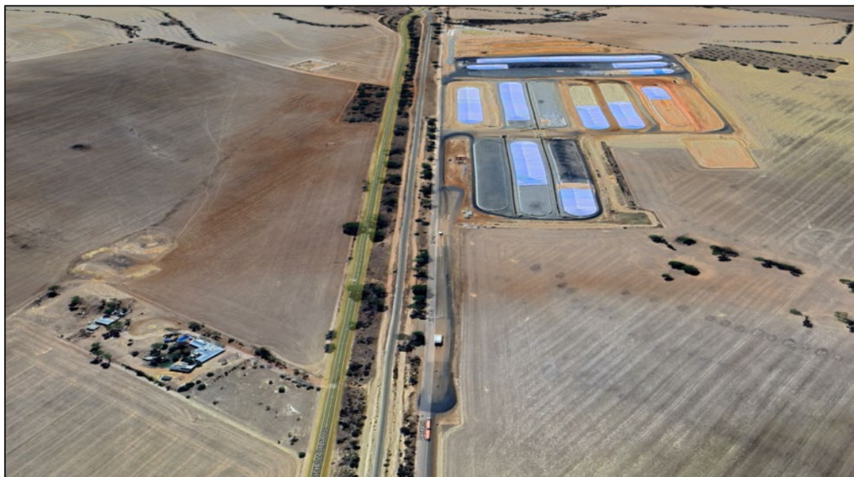
FIGURE 2 - OBLIQUE GOOGLE VIEW OF SITE
