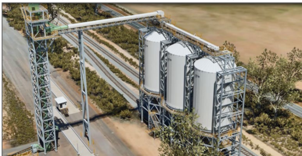
FIGURE 4 - PROPOSED OVER-RAIL BIN INFRASTRUCTURE
