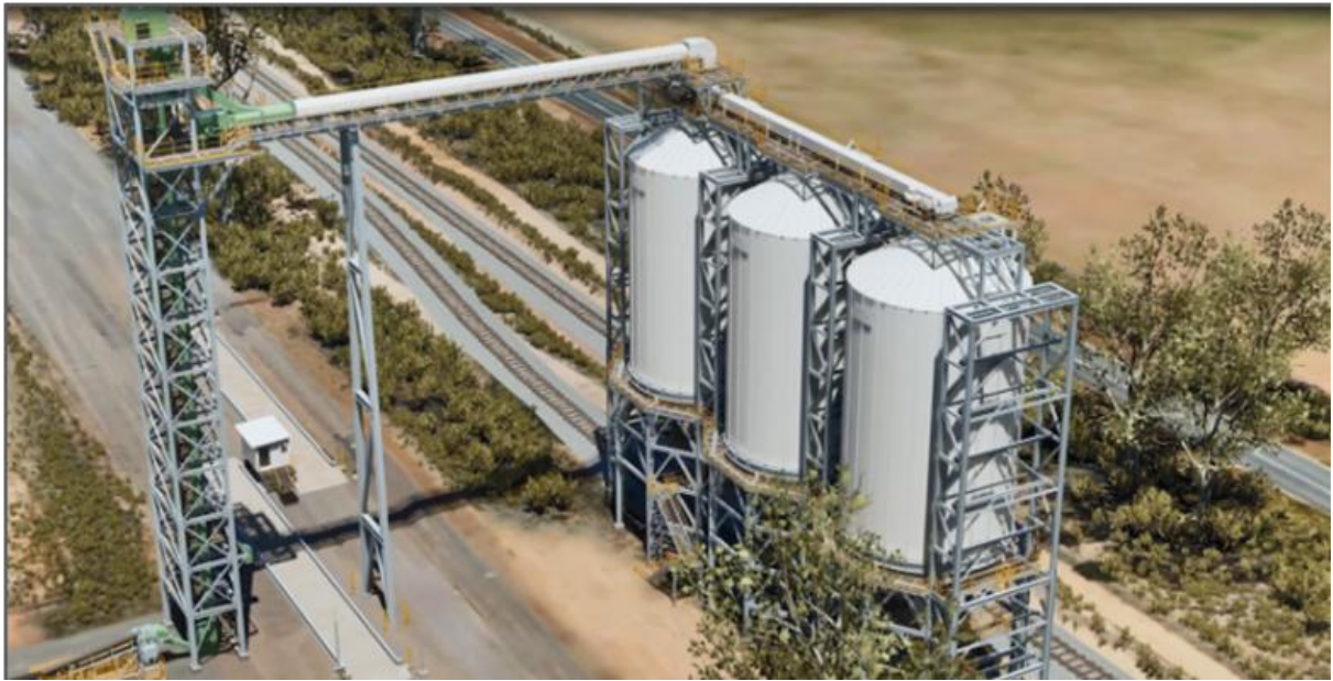
FIGURE 4 - PROPOSED OVER-RAIL BIN INFRASTRUCTURE
