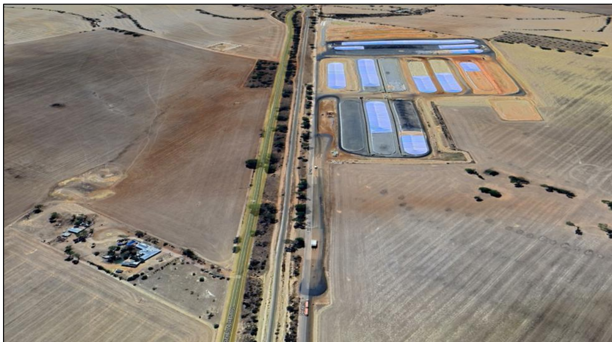
FIGURE 2 - OBLIQUE GOOGLE VIEW OF SITE
