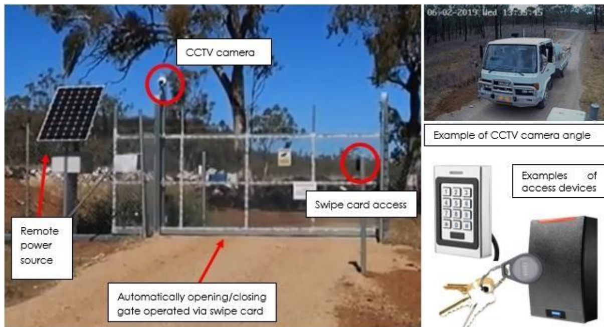
Figure 5.2 - Remote Access and Security System
