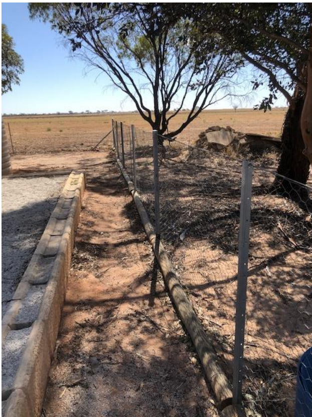
Front yard fence
